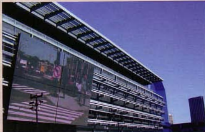
The igus E4/4 Energy Chain System with Chainflex cables supplies the giant LCD screens in Dallas, Texas with power and data
